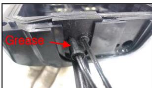
2. Inserting Flat Drop Gasket
