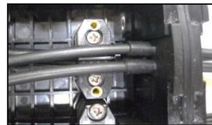
2. Inserting Drop Cable
