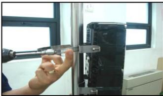
Pass the pole band through the hole of the hanger bracket and mount the closure on a pole.
