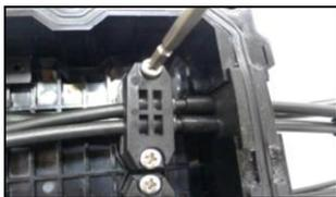
3. Fixing Cable Sheath
